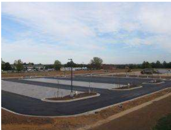
Figure 18 Permeable Surfaces
