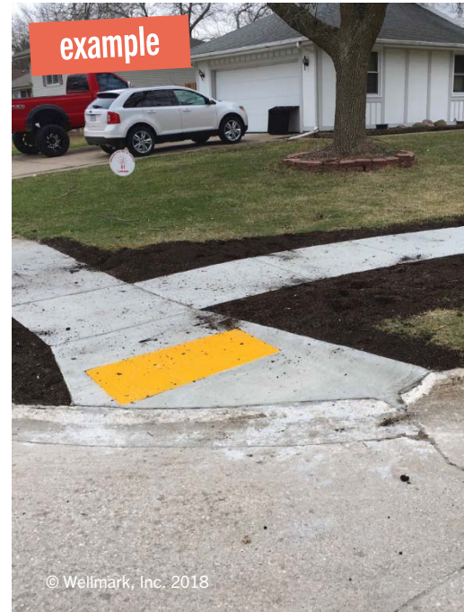
Example of a newly installed ADA-compliant curb ramp with yellow truncated domes for people with visual impairments to detect the edge of the crosswalk.
